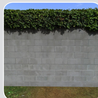
Prohibited material: cement block
