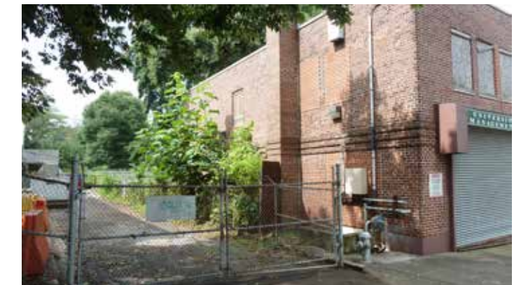
H. East elevation with fire exist, chimney and building utilities
