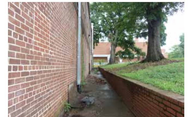
F. Building alley way on south
